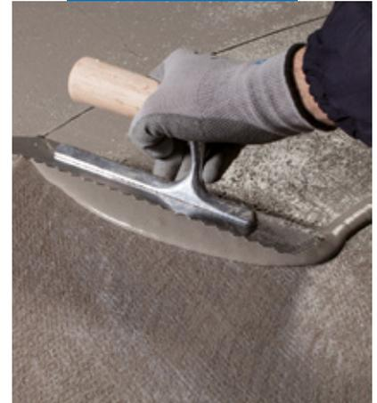
The second layer of Mapelastik Turbo over the first layer reinforced with Mapetex Sel
