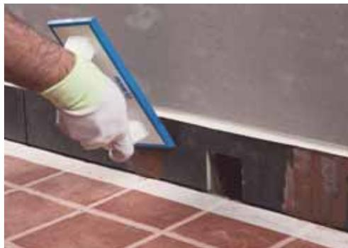
**12. Bond on the skirting boards and grout the vertical joints**
