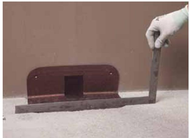
**1. Make a hole in the parapet and floor large enough to insert the Drain Front. Make sure it is perfectly level with the horizontal and vertical surfaces**
