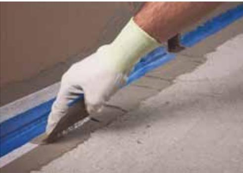
**9. Spread on a second layer of the specified MAPEI waterproofing product to completely cover the edges of the tape so they are sandwiched between the two layers of the cementitious mortar**
