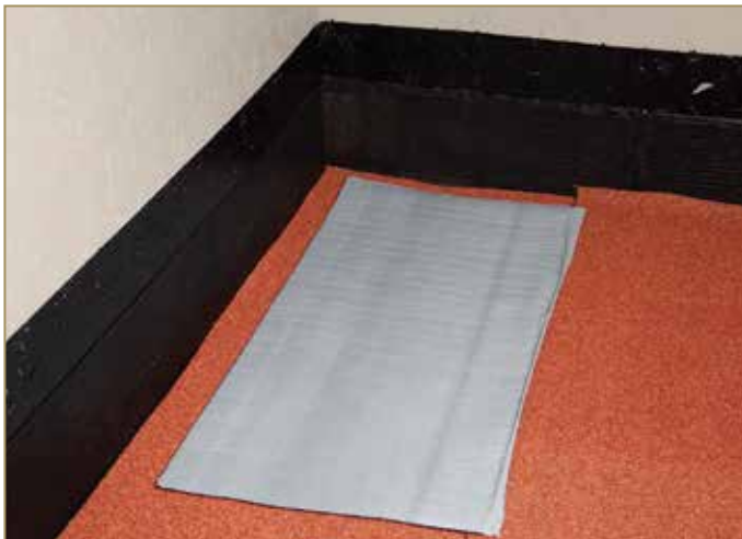
Figure 9.13: Preparing the vertical up-turn on granule surfaced membrane
