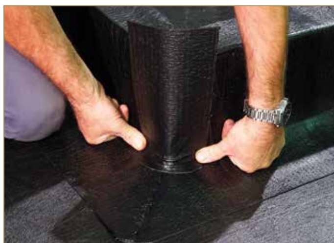
Figure 9.47: Positioning and gluing the closing patch
