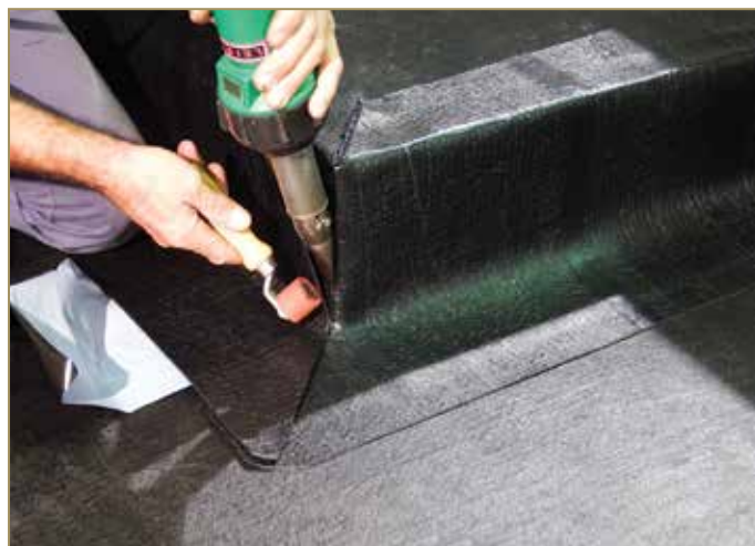
Figure 9.43: Up-turn at vertical welding
