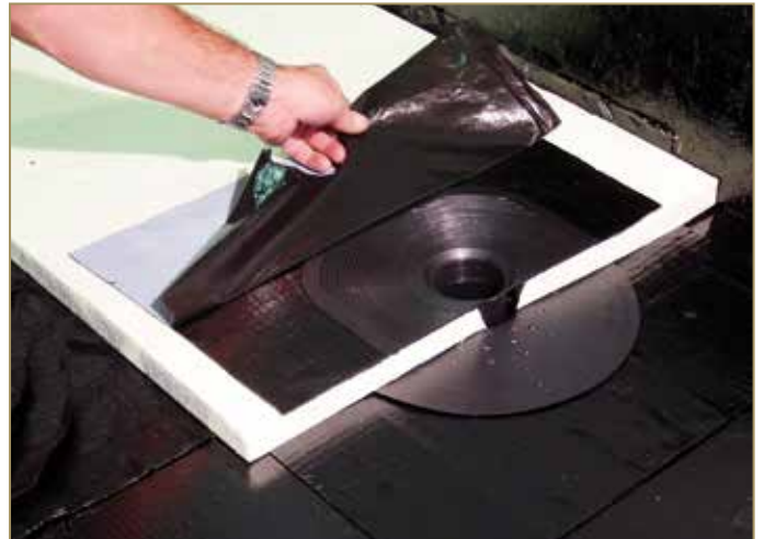
Figure 9.78: Removing the protective film
