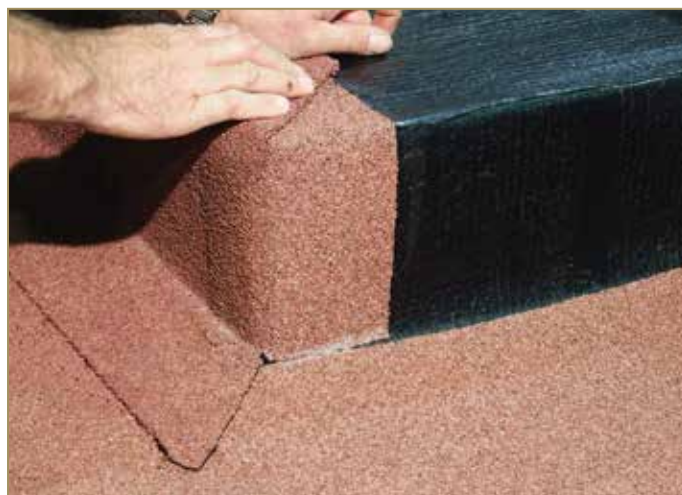
Figure 9.57: Folding the membrane on the upper edge
