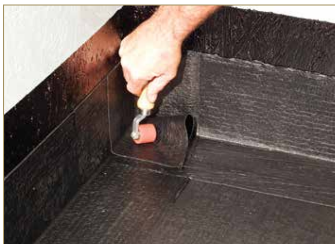
Figure 9.10: Horizontal gluing and rolling
