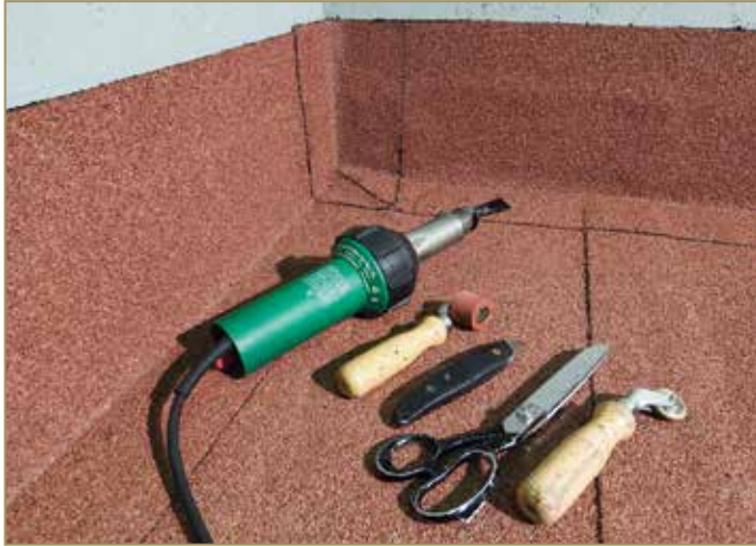
Figure 9.29: Corner and equipment used
