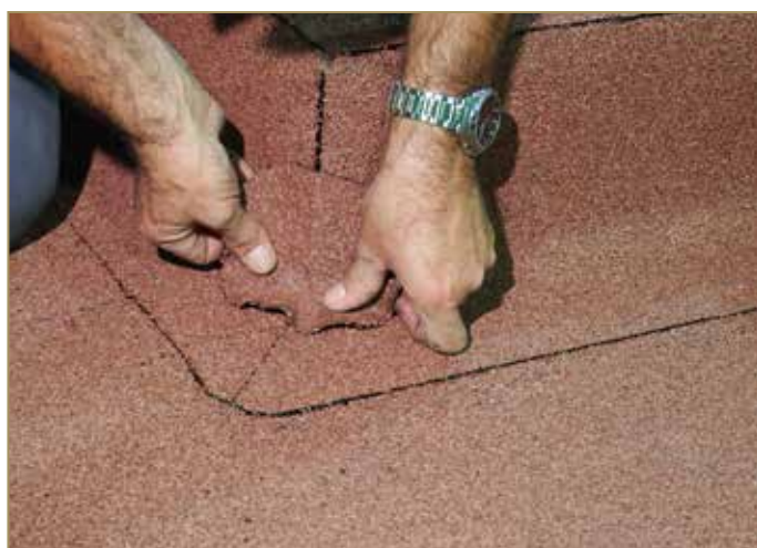
Figure 9.66: Preparing the closing membrane patch
