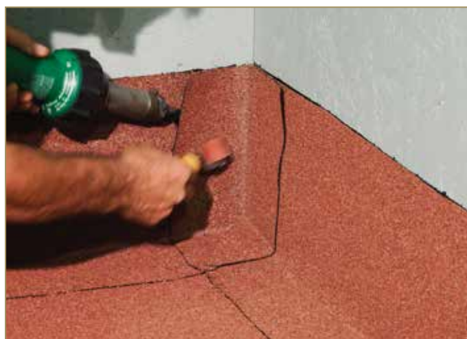
Figure 9.26: Welding the patch on the vertical wall
