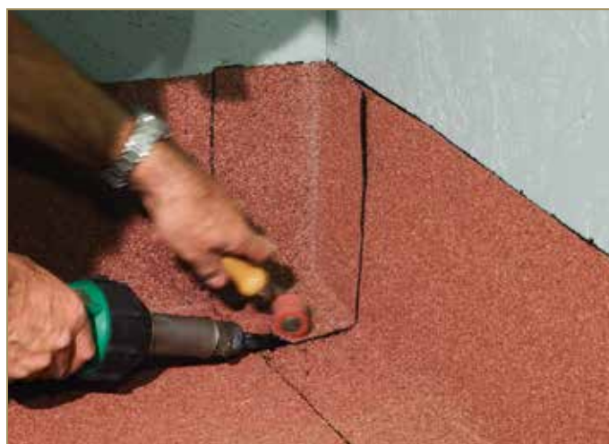
Figure 9.28: Hermetically closing and welding the corner
