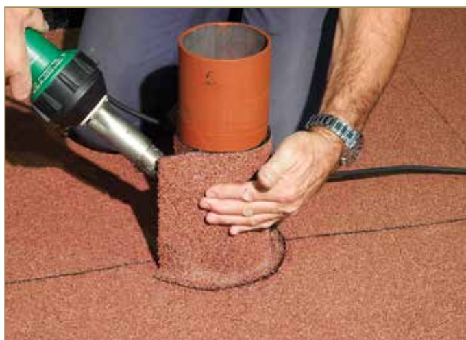
Figure 9.98: Welding the vertical part
