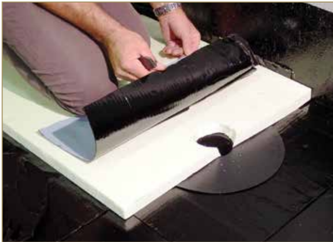
Figure 9.75: Positioning the membrane under the outlet
