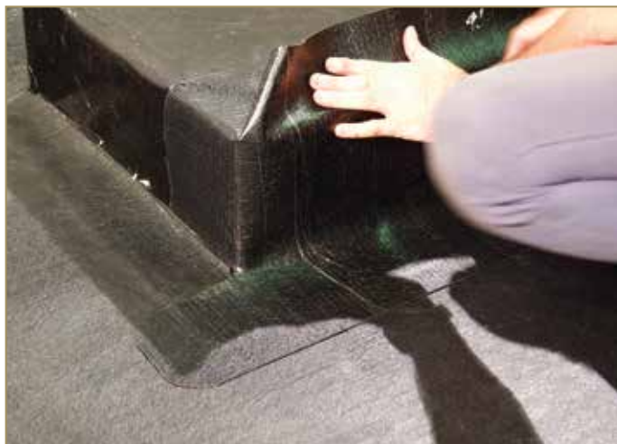
Figure 9.38: Folding the membrane on the upper edge
