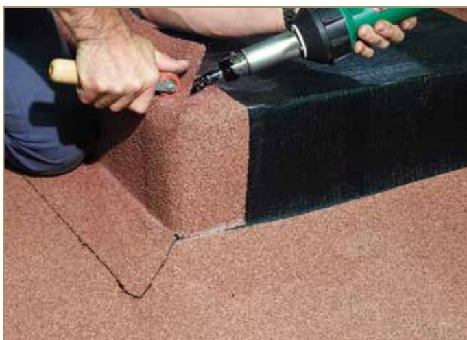
Figure 9.58: Hermetically closing and welding the corner
