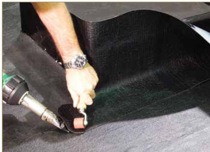
Figure 9.37: Welding the overlap on the flat surface
