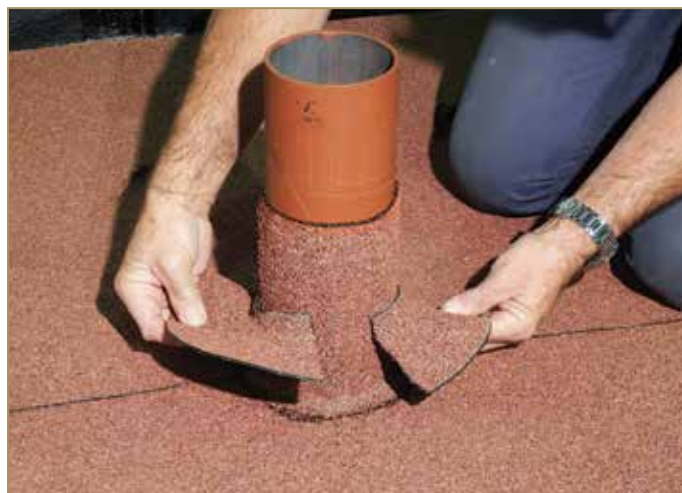
Figure 9.100: Positioning the covering patch
