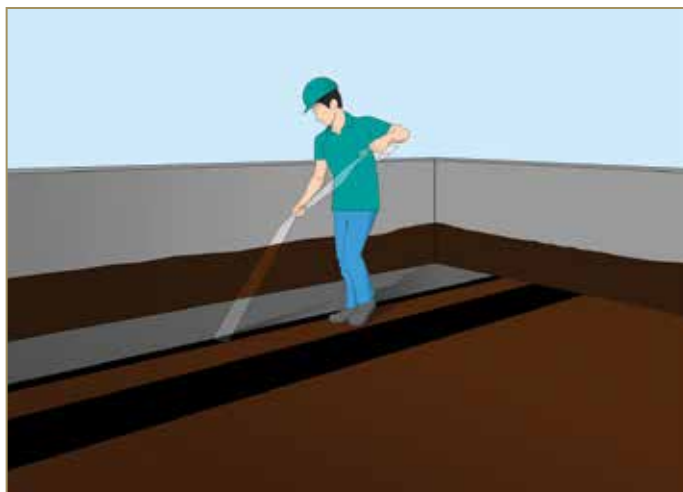
Figure 7.13: Remove the protective film on the side sedge of the adjacent membrane
