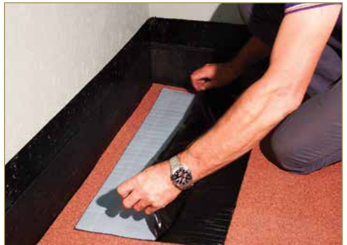
Figure 9.14: Partially removing the protective film
