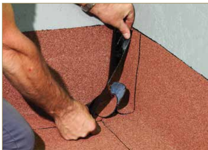
Figure 9.25: First gluing phase of the membrane patch
