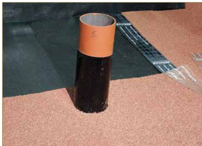
Figure 9.90: Removing the protective film and gluing the second waterproof layer
