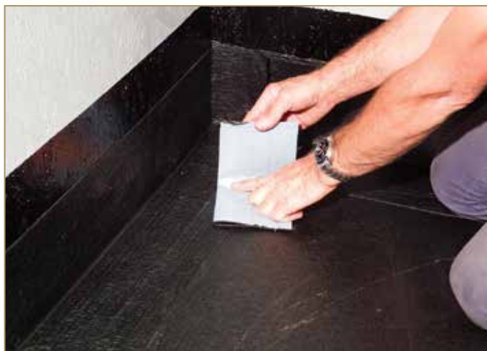
Figure 9.5: Folding the patch of membrane into 4 parts
