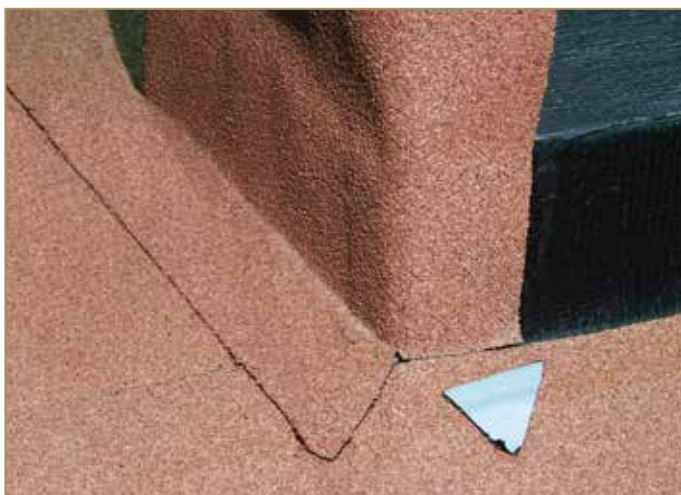
Figure 9.56: Trimming and cutting off the excess membrane (triangle)
