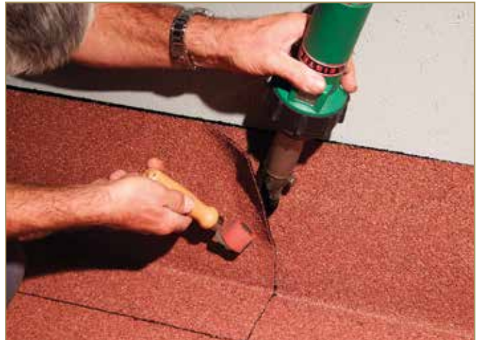
Figure 9.32: Up-turn at vertical welding
