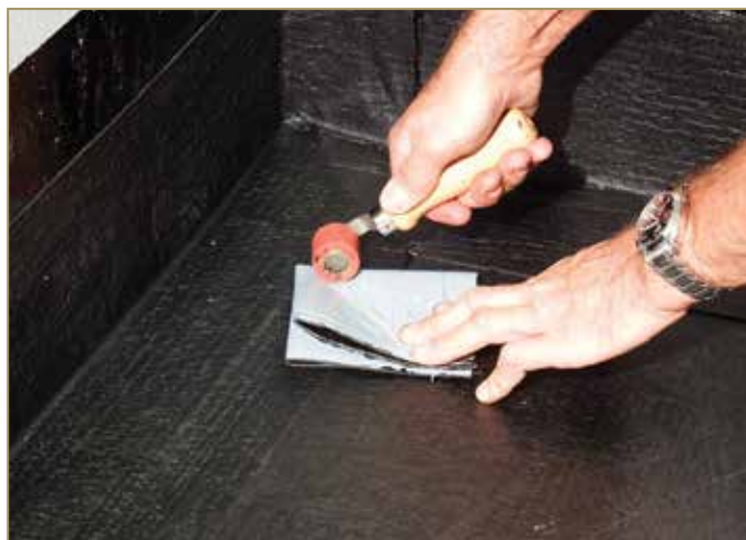
Figure 9.6: Rolling to mark the 4 corner portions
