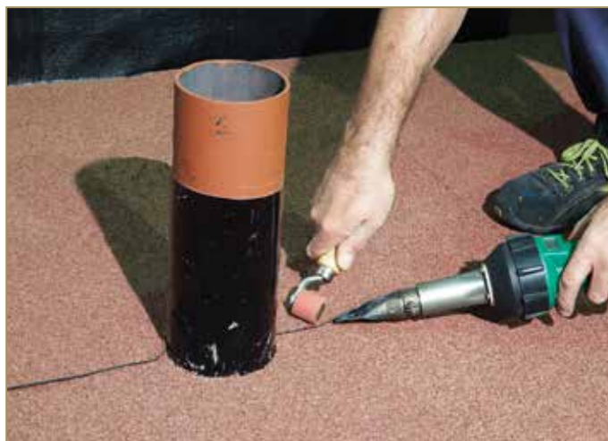
Figure 9.94: Closing weld of the overlap at the beginning of the roll
