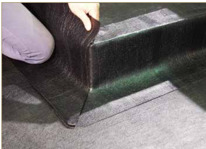
Figure 9.42: Gluing on the vertical wall of the up-turn
