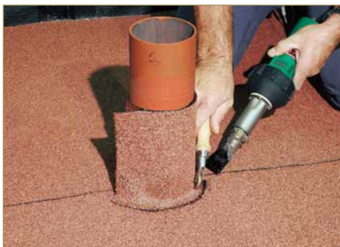
Figure 9.97: Welding and rolling the up-turn foot
