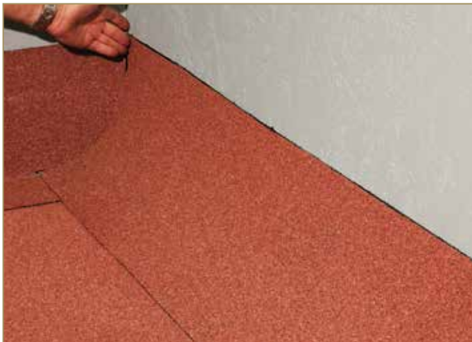
Figure 9.19: Preparing the vertical up-turn on the adjacent wall
