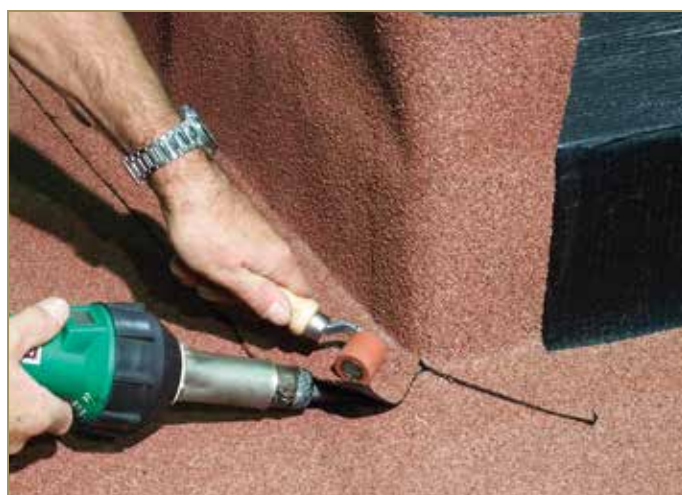
Figure 9.55: Welding the overlap on the flat surface
