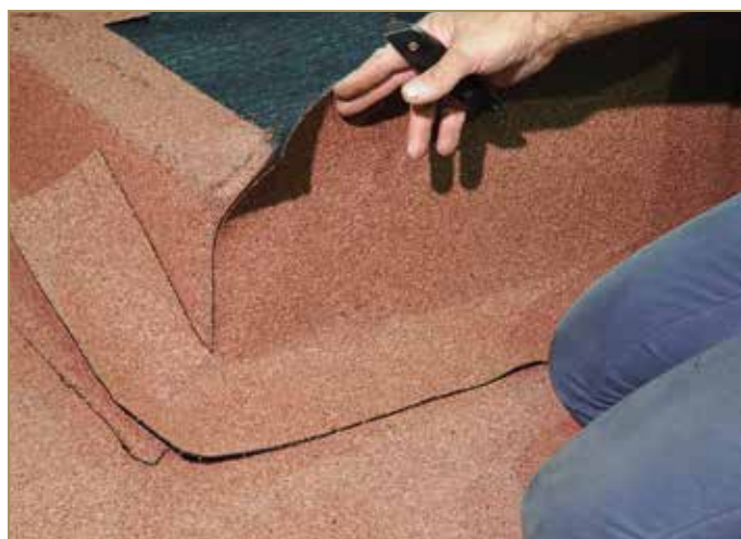
Figure 9.59: Preparing and gluing the adjacent vertical up-turn
