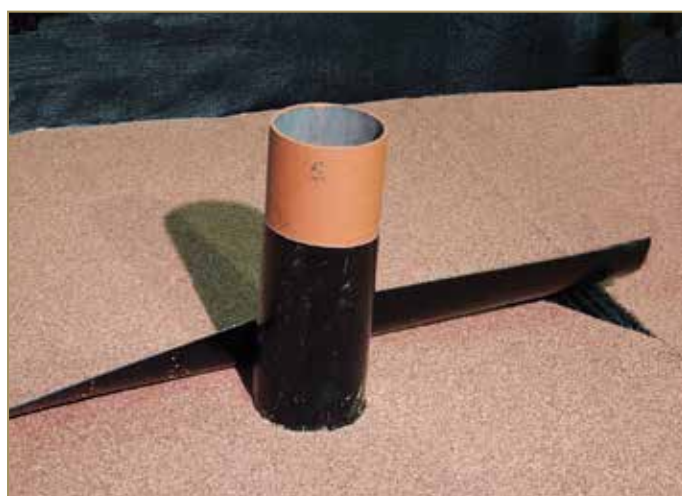
Figure 9.92: Removing the protective films and gluing the membrane
