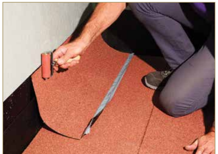
Figure 9.16: Rolling the top part
