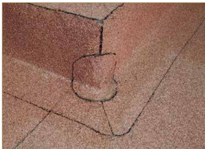
Figure 9.68: Finished external corners
