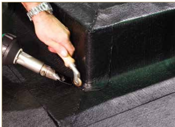
Figure 9.49: Welding the patch on the flat surface
