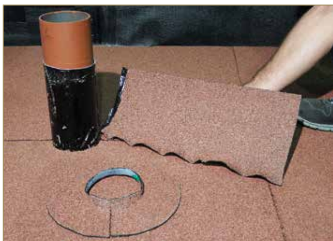
Figure 9.95: Preparing the elements to line the tube
