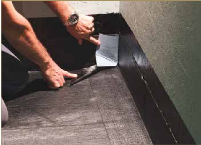
Figure 9.1: Preparation of the internal corner
