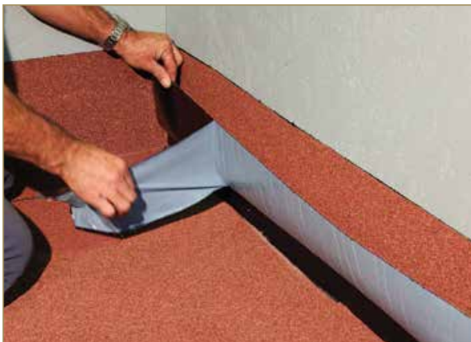
Figure 9.21: Total removal of the release film
