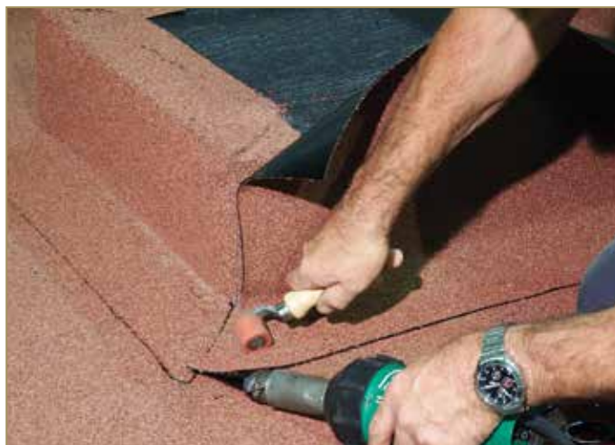
Figure 9.61: Welding the overlap on the flat surface
