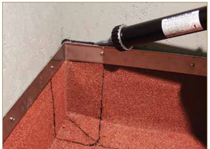
Figure 9.34: Sealing using POLYDETAIL MS
