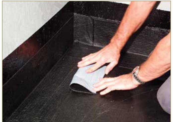
Figure 9.4: Cutting a 20x20 cm patch of membrane
