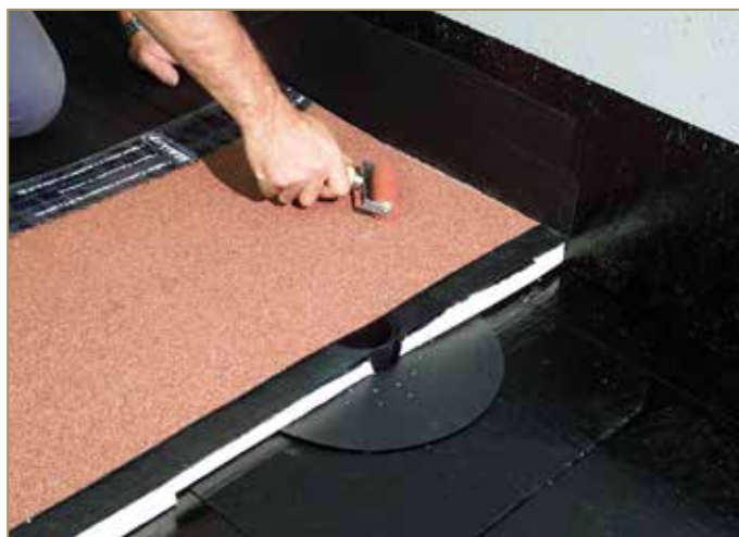
Figure 9.84: Rolling and gluing on the flat surface
