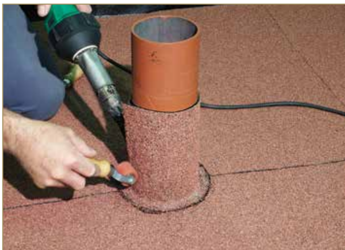
Figure 9.99: Welding the overlap on the vertical tube
