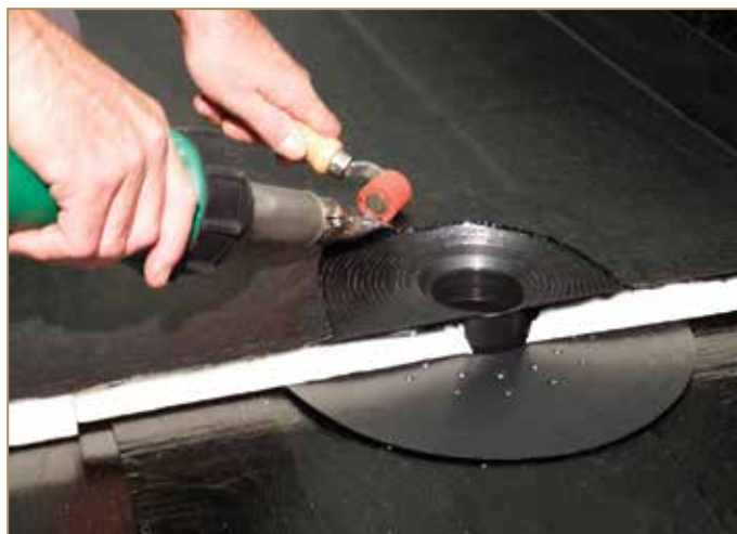
Figure 9.82: Closing weld of the first layer on outlet
