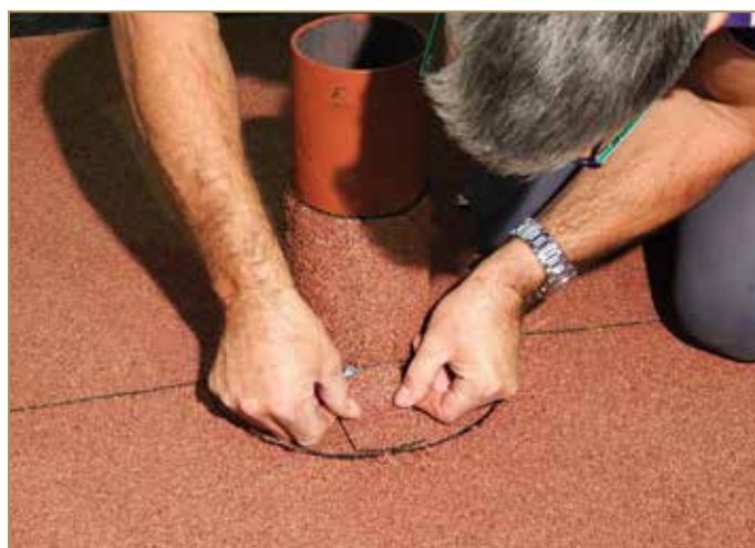
Figure 9.102: Positioning the closing patch
