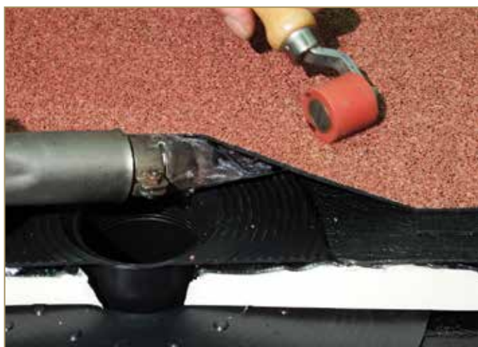
Figure 9.85: Closing weld of the second layer on outlet
