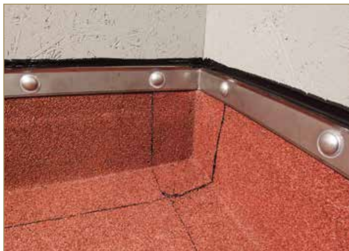
Figure 9.35: Completed internal corner with profile and studs
