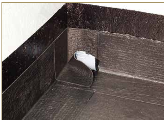
Figure 9.8: Application and gluing of the patch on the vertical wall
