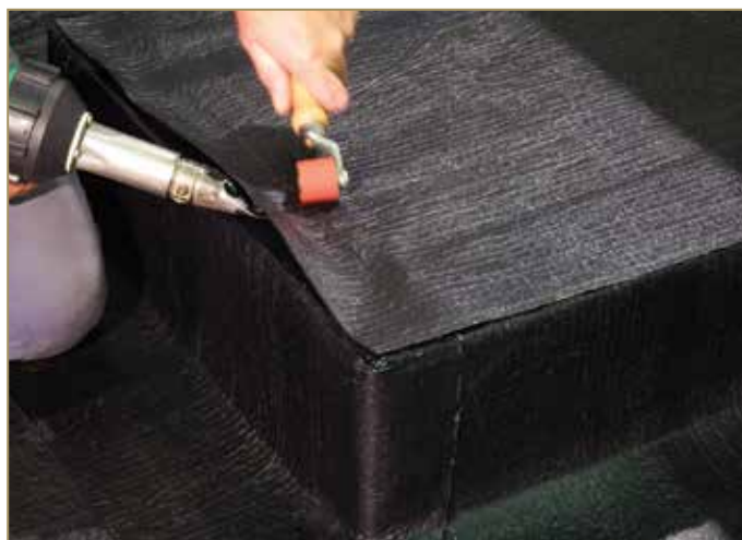
Figure 9.51: Closing weld of the top of the protruding structure
