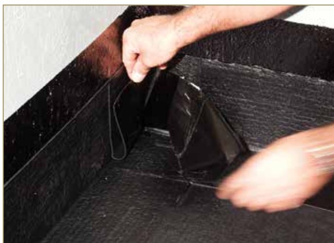
Figure 9.9: Removing the protective film
