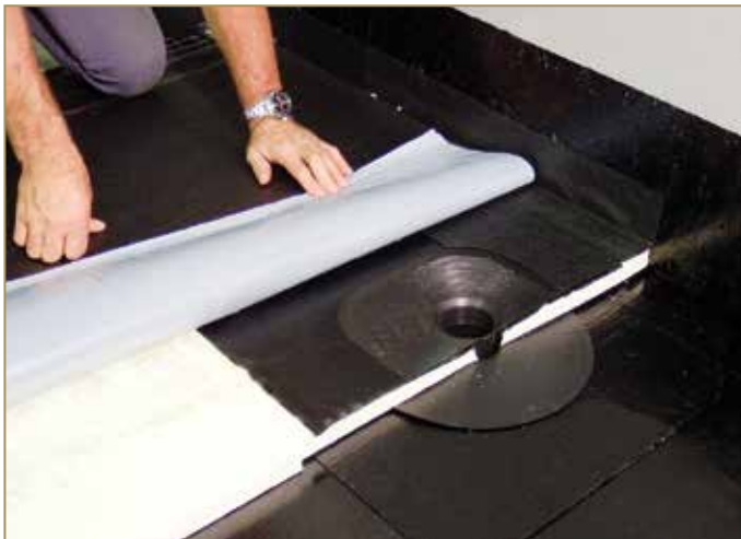
Figure 9.79: Positioning the first waterproof layer
