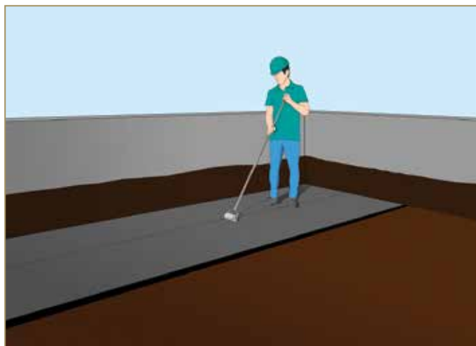
Figure 7.16: Use a roller to ensure a proper seal at the overlaps
