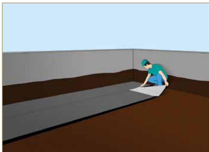
Figure 7.9: Check the position of the membrane and the side overlaps with the adjacent sheets
