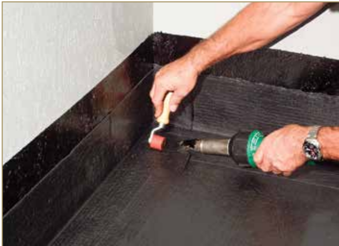
Figure 9.3: Flat welding
