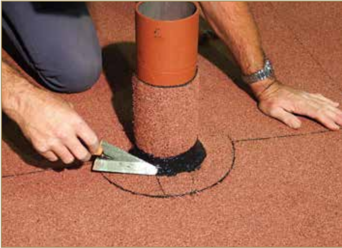
Figure 9.105: Levelling the POLYDETAIL MS
