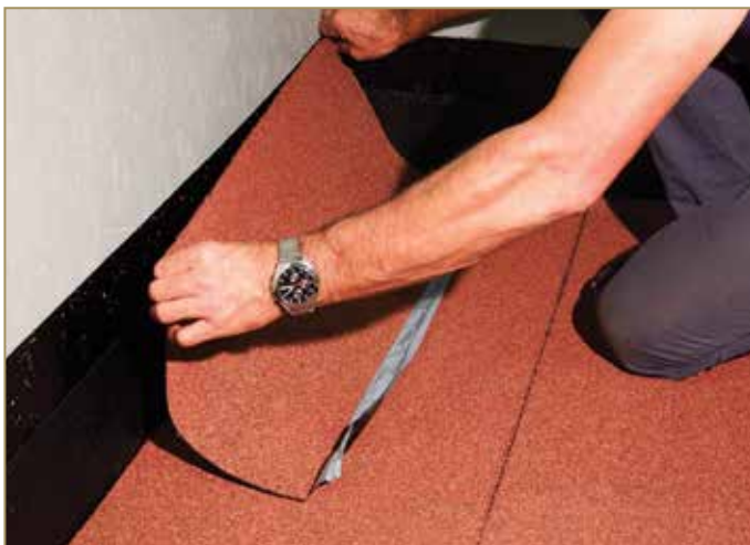
Figure 9.15: Positioning and gluing on the vertical up-turn
