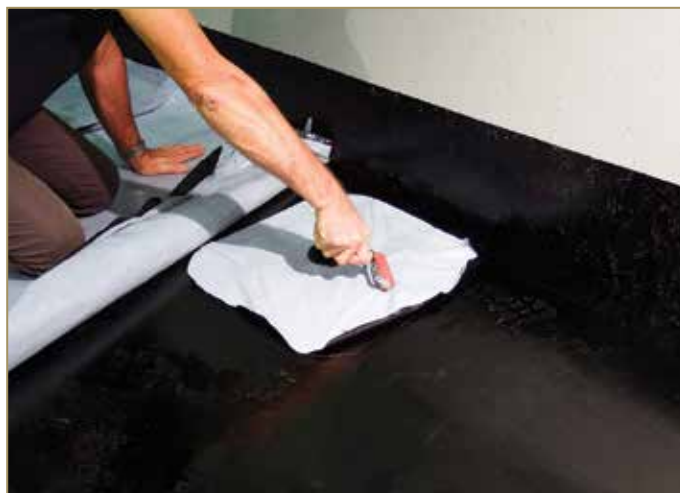
Figure 9.72: Replacing the protective film and rolling to glue outlet
