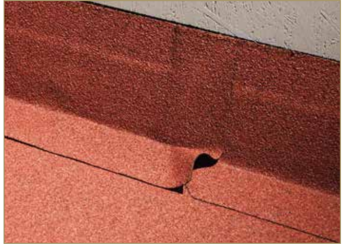
Figure 9.30: Overlap of two adjacent vertical up-turn
