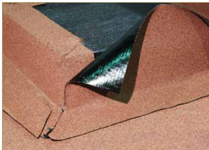
Figure 9.60: Cut at 45° of the overlapping part on the surface
