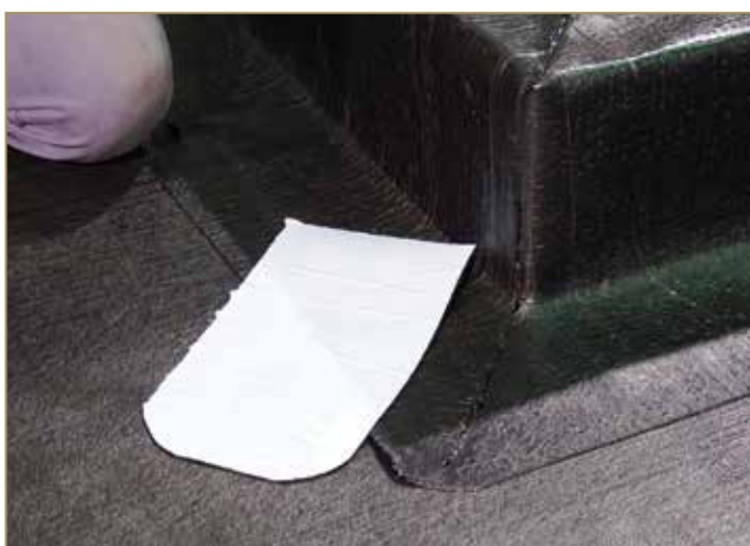
Figure 9.46: Preparing the shaped patch of membrane for the corner
