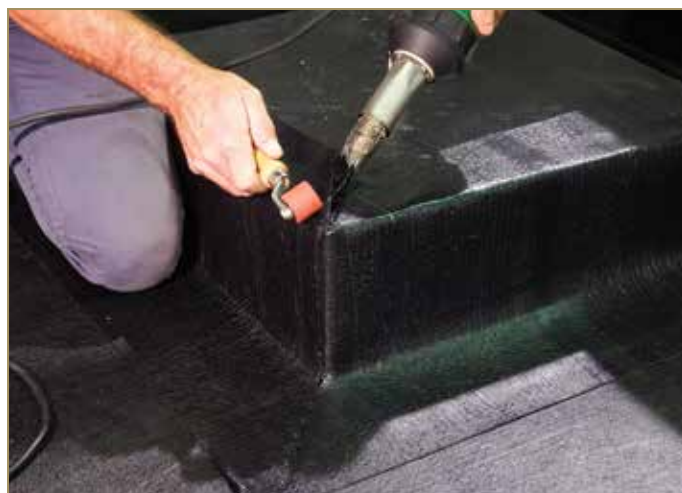
Figure 9.45: Welding the upper corner
