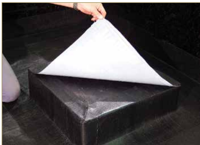
Figure 9.50: Preparing the top of the protruding structure
