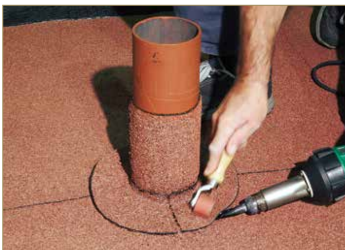
Figure 9.101: Welding the covering patch on the flat surface
