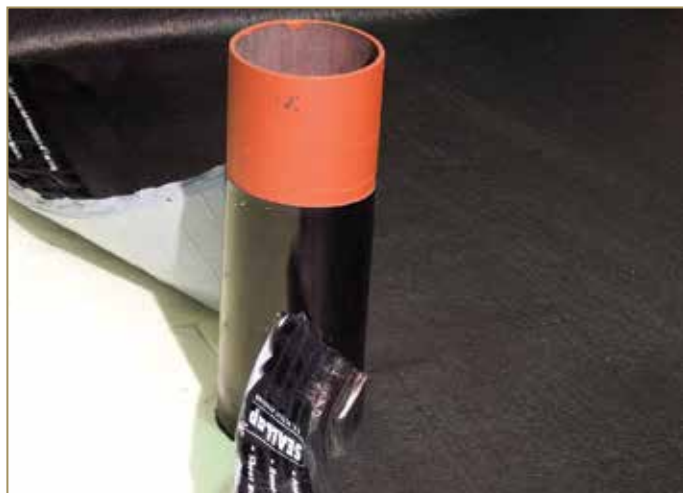
Figure 9.87: Positioning and cutting the first waterproof layer
