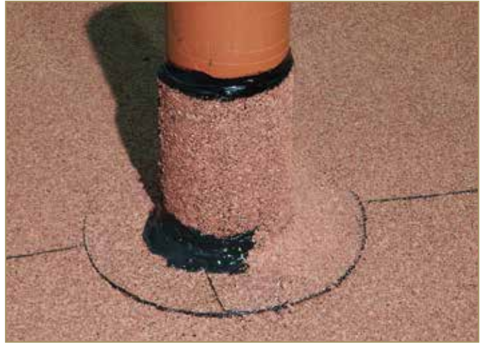
Figure 9.106: Top seal and aesthetic finish of the seal with slate chippings
