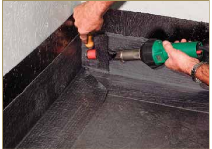
Figure 9.2: Up-turn vertical welding
