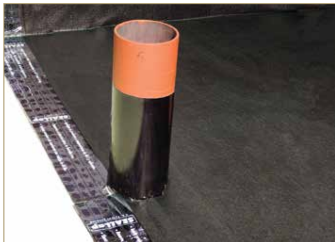
Figure 9.88: Removing the protective film and gluing the first layer
