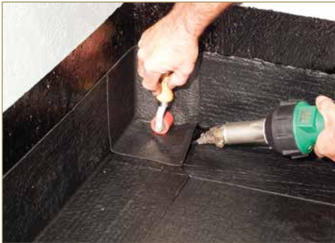
Figure 9.11: Hermetically closing and welding the corner
