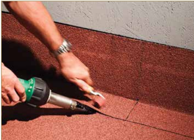
Figure 9.31: Welding the overlap on the flat surface
