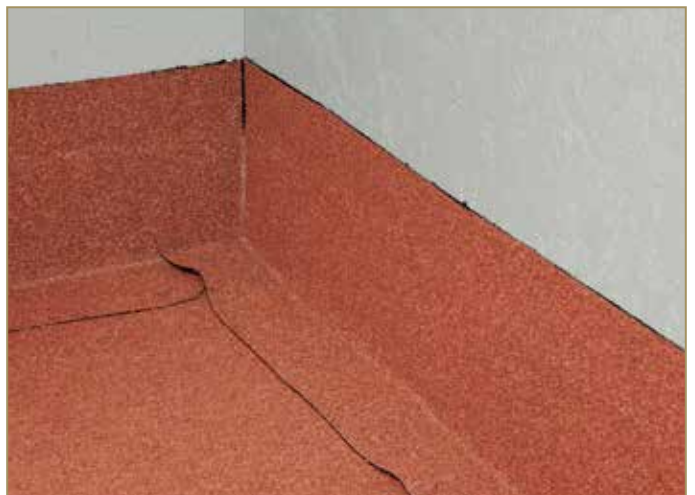
Figure 9.22: Vertical up-turn adhered to the wall
