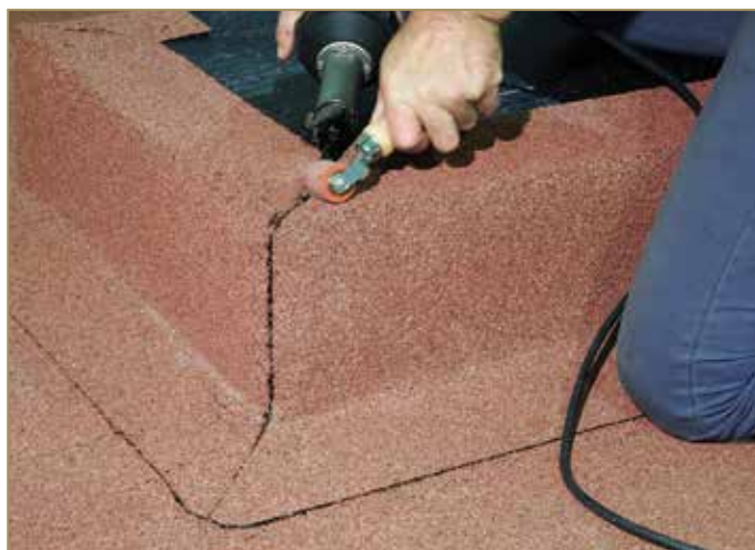
Figure 9.63: Welding the upper corner
