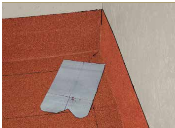
Figure 9.24: Preparing the shaped patch of membrane for the corner
