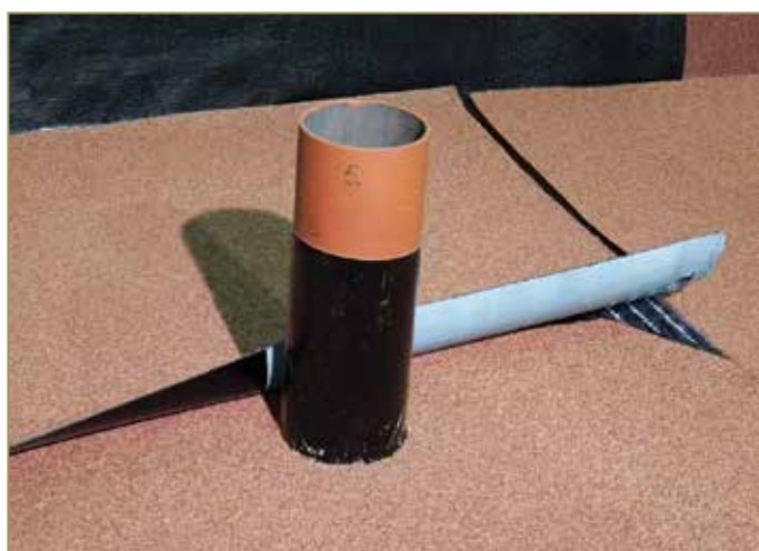
Figure 9.91: Positioning the adjacent membrane and preparing the overlap at the beginning of the roll
