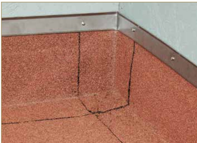
Figure 9.33: Fixing the termination profile to the wall
