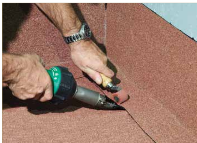
Figure 9.23: Welding the overlap on the flat surface
