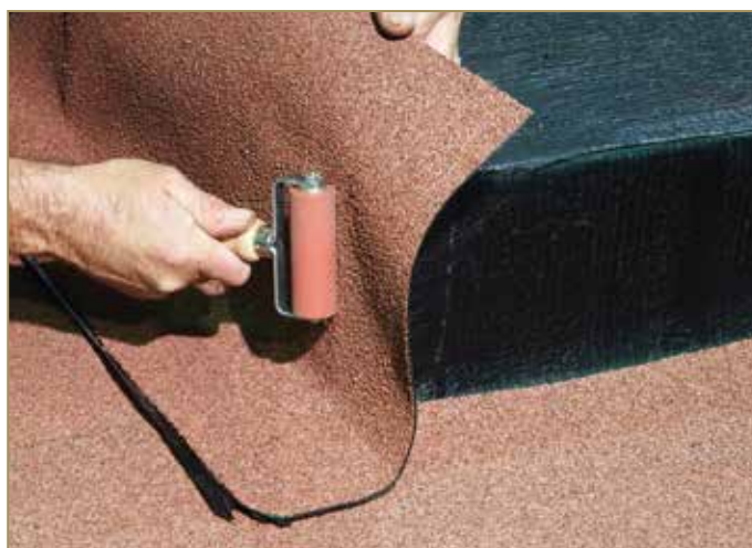
Figure 9.53: Gluing and rolling the vertical up-turn
