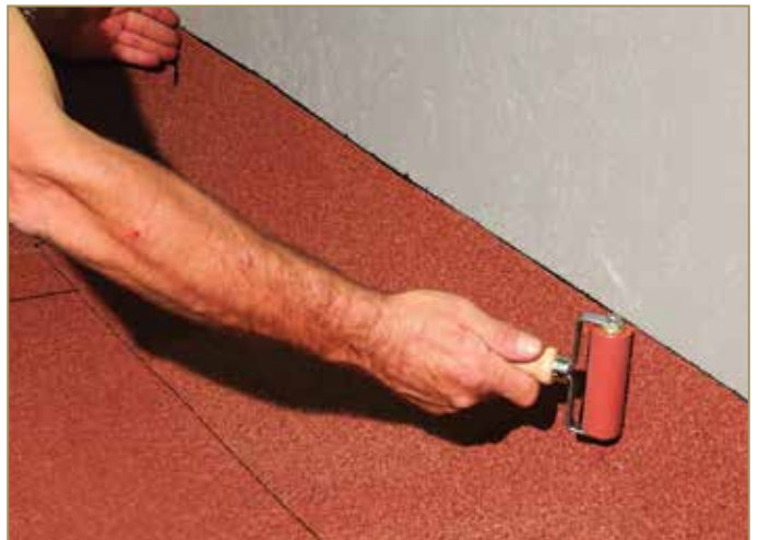
Figure 9.20: Rolling the vertical detail
