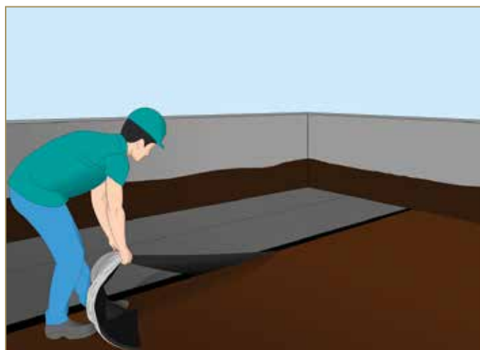
Figure 7.10: Remove part of the release mono-silicone protective film on the bottom side, to adhere the first half of the membrane
