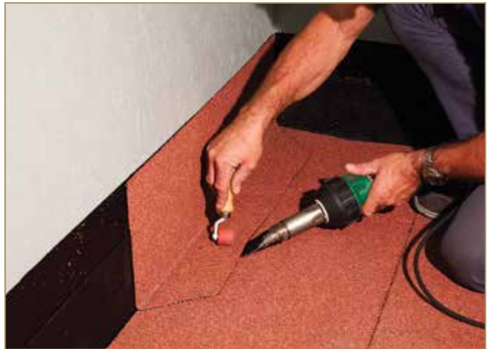
Figure 9.18: Welding the overlap on the flat surface
