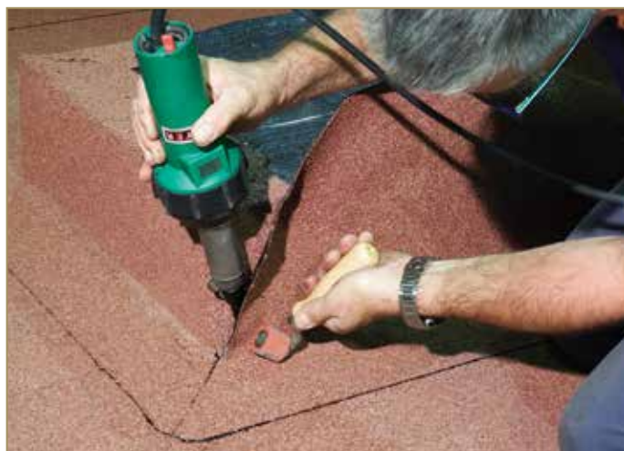
Figure 9.62: Welding the vertical overlap
