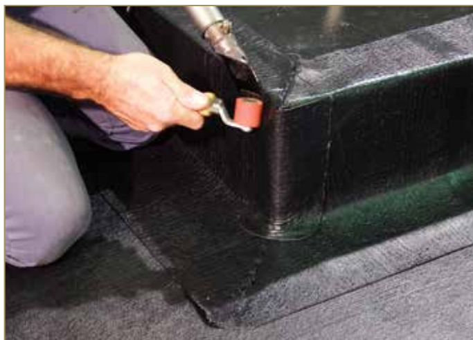
Figure 9.48: Welding the patch on the vertical wall
