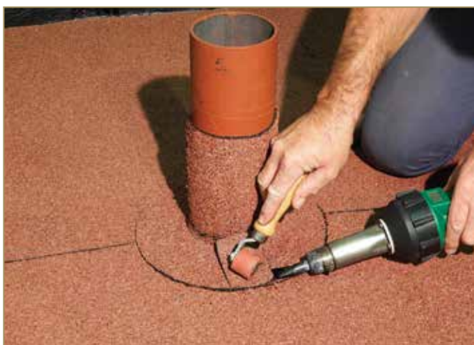
Figure 9.103: Closing weld of the patch cut
