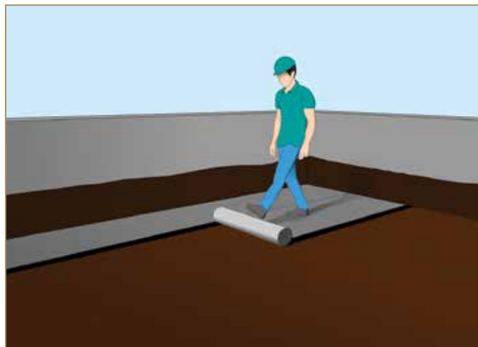
Figure 7.8: Unroll the membrane in its final position
