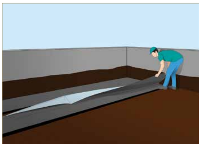
Figure 7.11: Fold over the loose half of the membrane
