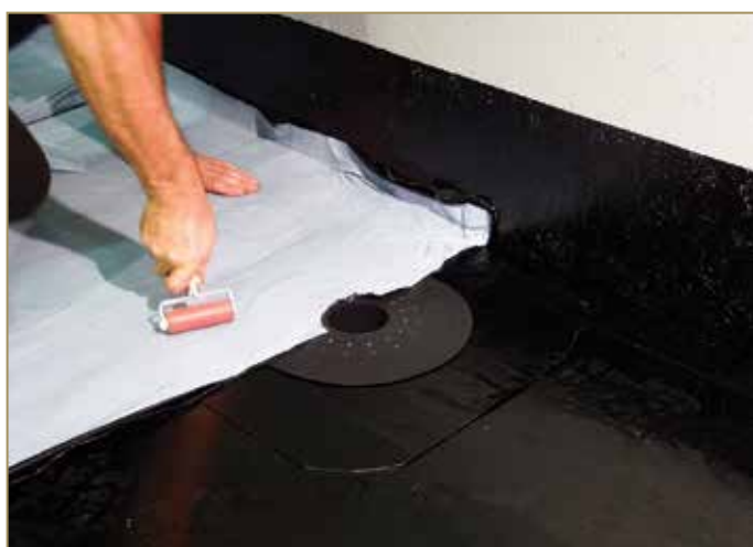
Figure 9.73: Positioning the ADESO ® vapour barrier and rolling
