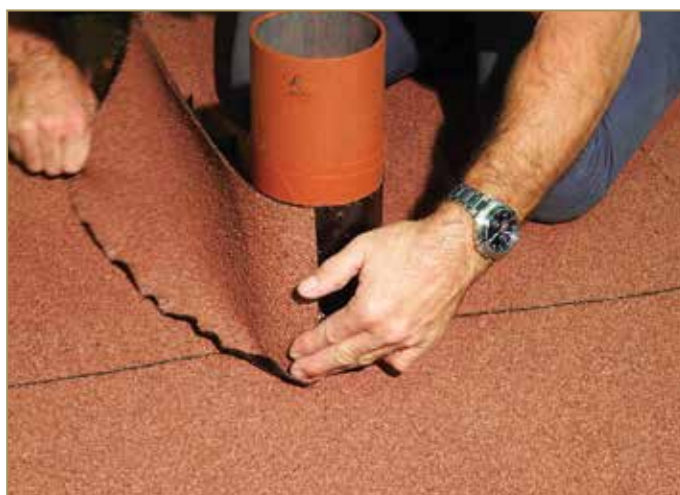
Figure 9.96: Gluing the vertical up-turn on the tube
