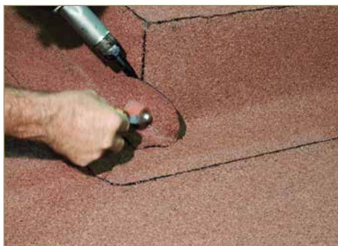
Figure 9.67: Welding the patch
