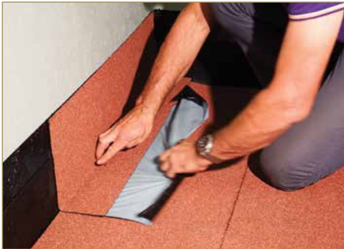
Figure 9.17: Removing the protective film
