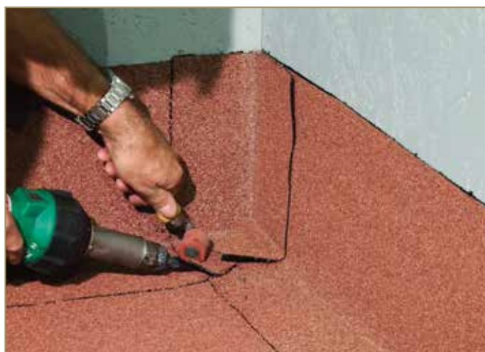
Figure 9.27: Welding the patch overlap on the flat surface
