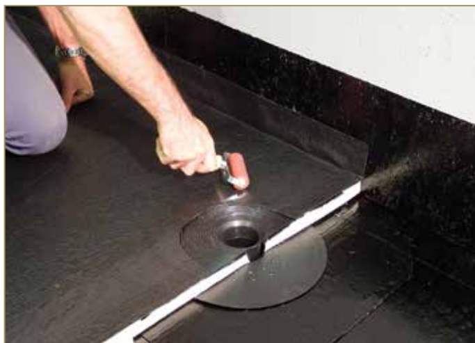
Figure 9.81: Membrane gluing and rolling
