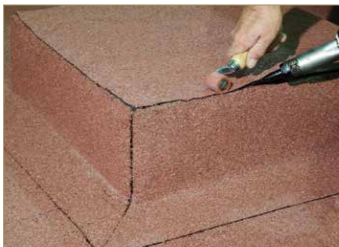
Figure 9.65: Welding the upper edge
