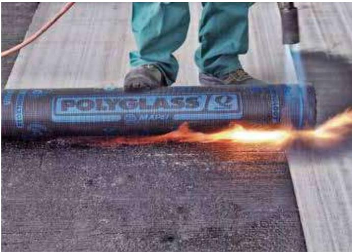
Membrane from Reoxthene line being torched on.
