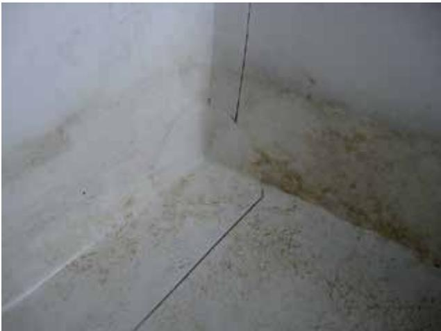
After two years lining the growing boxes, the MAPEPLAN T B lining proves perfectly undamaged and features no signs of piercing or deterioration either on the surface or along the main and detail welding.
