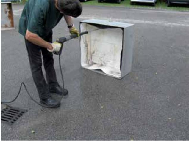
After two years, the vegetation is removed along with the soil and the root-resistant waterproofing membrane is cleaned with a water blaster.
