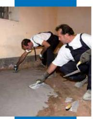
Application of the first layer of Planitop HDM Restauro by trowel on the outer face of a vaulted ceiling
