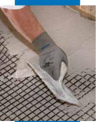
Application of the second layer of Planitop HDM Restauro by trowel on the outer face of a vaulted ceiling to cover the Mapegrid G 220 with an even coat
