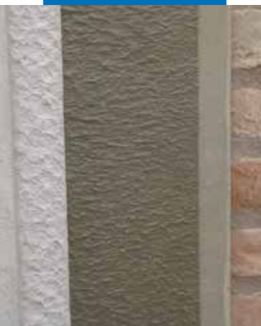
Application of PoroMap Rinzafo Plus on Mapelastic Foundation for creating anti-condensation cycle
