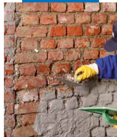
Application of PoroMap Rinzafo Plus with a trowel
