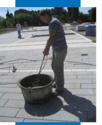
Mix Mapestone PFS 2 Visco with water only using a mixing attachment or cement mixer
