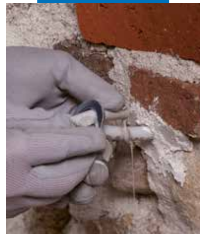
Closing the injection tubes
