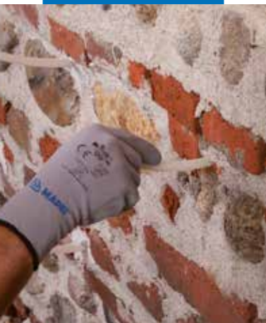
Positioning the small injection tubes
