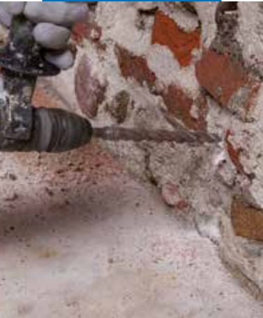
Drilling the holes
