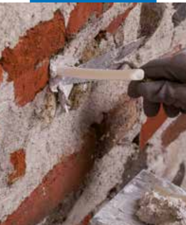
Fastening the small injection tubes in place
