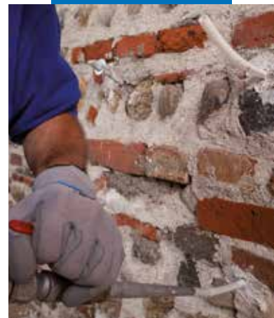
Injection of MapeWall Inject & Consolidate
