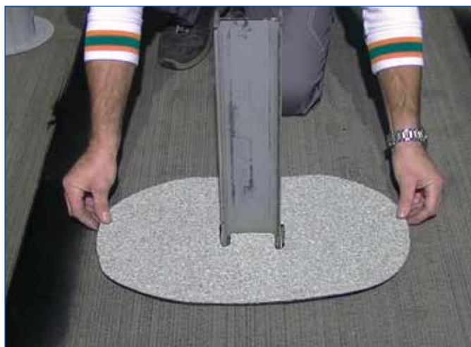
FIGURE 7 - Application of patch of mineral membrane
