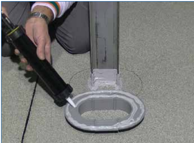
FIGURE 4 - Application of the POLYSEALANT CARTRIDGE adhesive sealant
