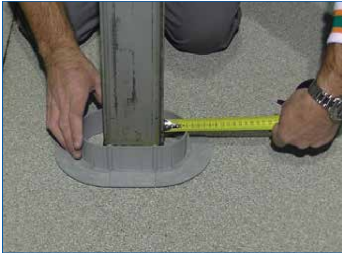
FIGURE 3 - Positioning of the formwork
