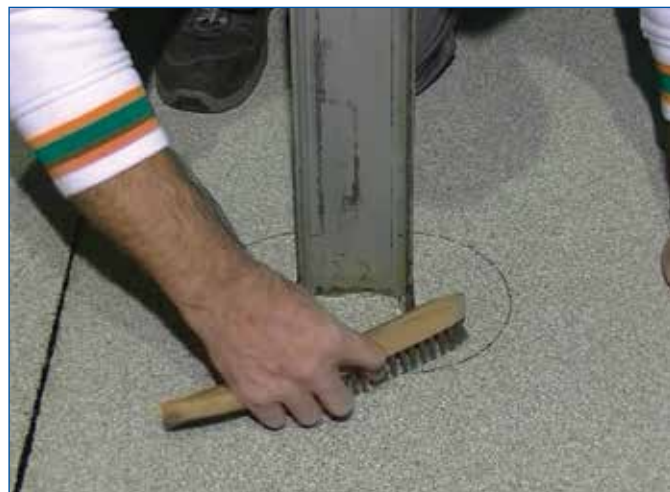
FIGURE 2 - Preparing the surfaces
