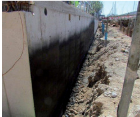
Foundation wall waterproofed with Plastimul 2K Reactive
